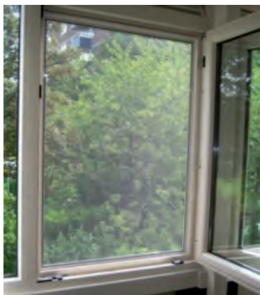
Hor in raamopening (bron: rendementbouw.nl)
