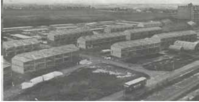
Picture 5c.13 First houses are built. Source: Rotterdams Dagblad
