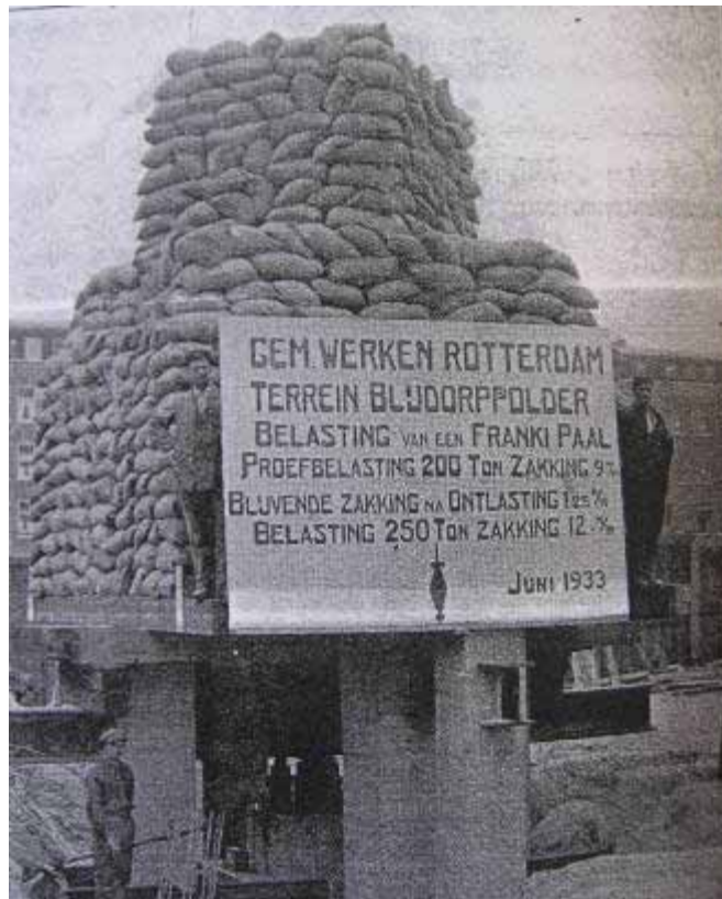
Picture 5.7 Tests with the Franki piles in Blijdorp 1933 Source: De Ingenieur 1934
